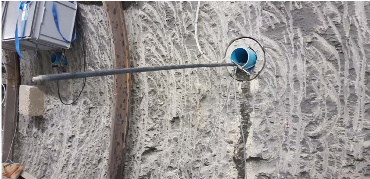
Figure 7-3: Installation of the transmitter in the middle access borehole
