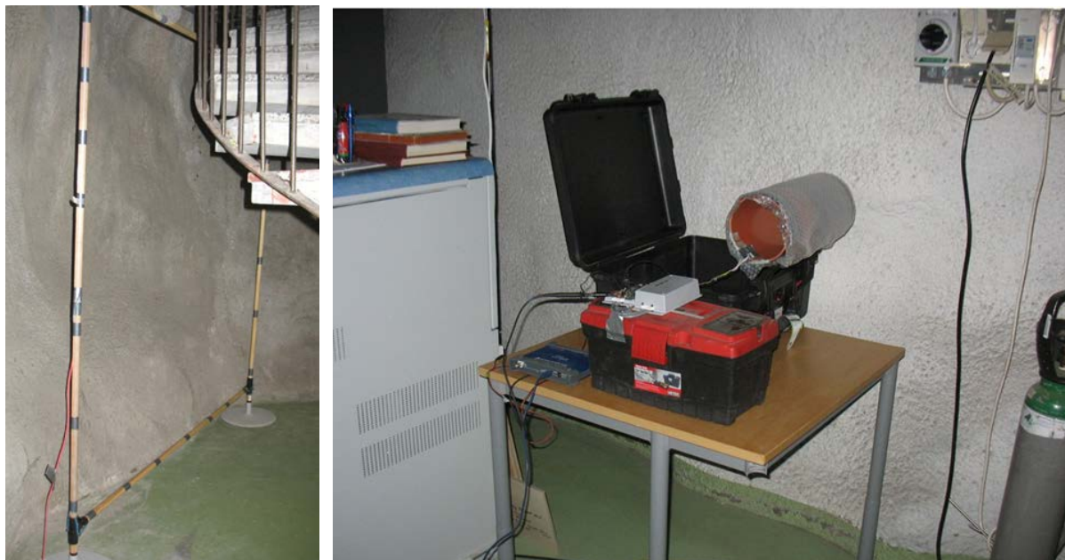
Figure 6-9. The pilot system in co-axial antenna configuration in the bedrock cave at VTT Otaniemi. The leftmost photo presents the reader antenna and the rightmost photo the sensor part.
