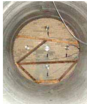
Completed bentonite buffer
