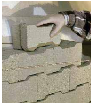
Bentonite buffer construction
