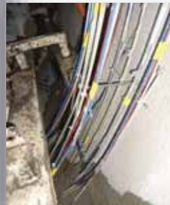
OF measurements in concrete lining
