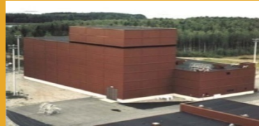
Interim storage of spent nuclear fuel
