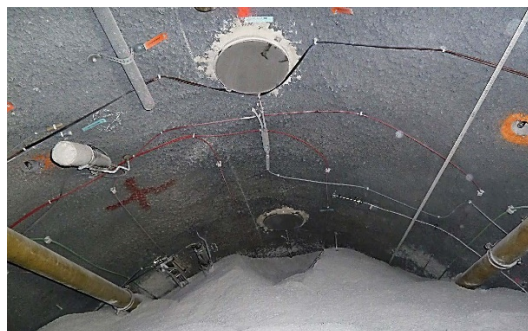
Figure 65: Behind the concrete plug
