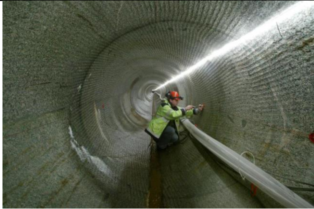
Figure 1. The 95 m drift at Äspö HRL, \varnothing 1.85 m
