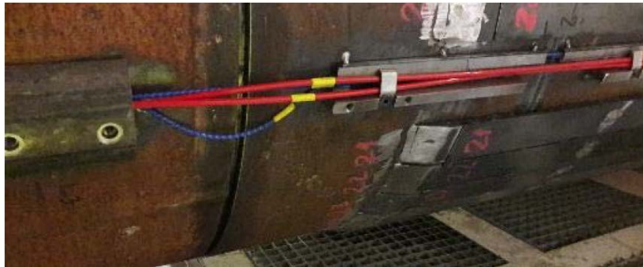
Figure 25: On site longitudinal of installation with two different configurations of fixation for SSV9 cables (blue)
