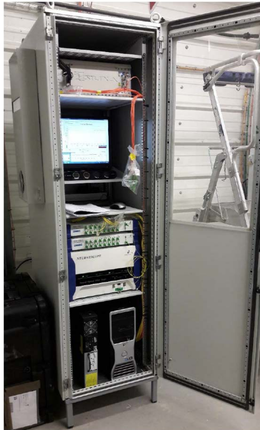
Figure 33. Dust-proof box with monitoring system components
