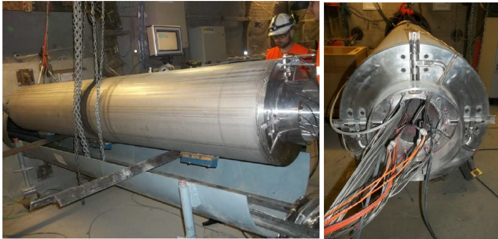
Figure 42: View of a heater element during installation on ALC1604 (left) – View of a heater/sleeve distance variation sensor section (right)
