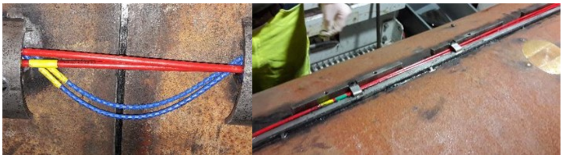
Figure 26: Photos of the longitudinal OFS cable installed at the top (right) and the over length for installation management (left)
